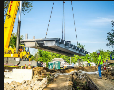
NEW ROADWAY BRIDGES
